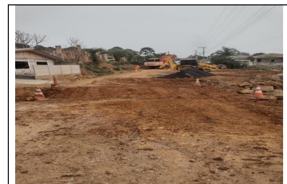
10 – RUA NADIR OSVALDO MIKETEN – REATERRO DE VALA
